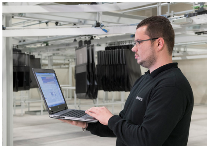
Operations and maintenance staff use software with a current state view that includes actionable information.
