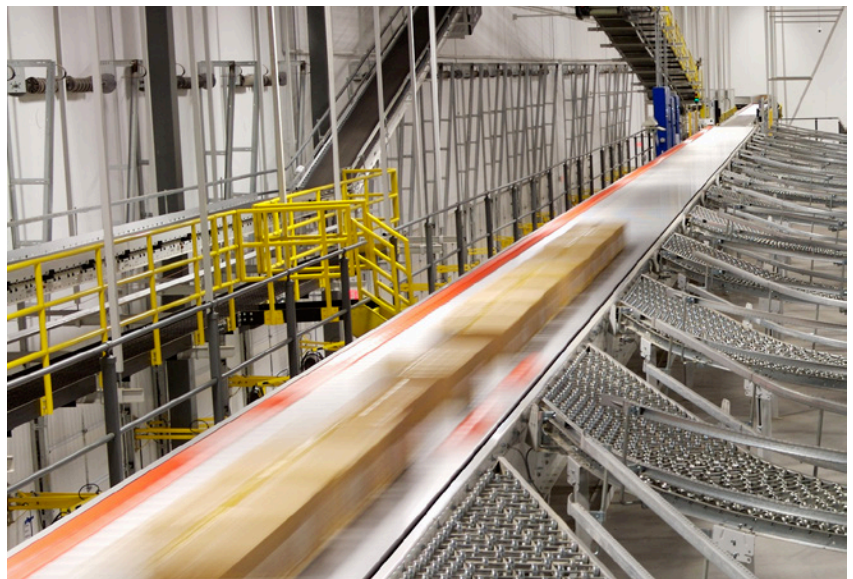
The Sliding Shoe Sorter accommodates a door-per-store shipping operation.
