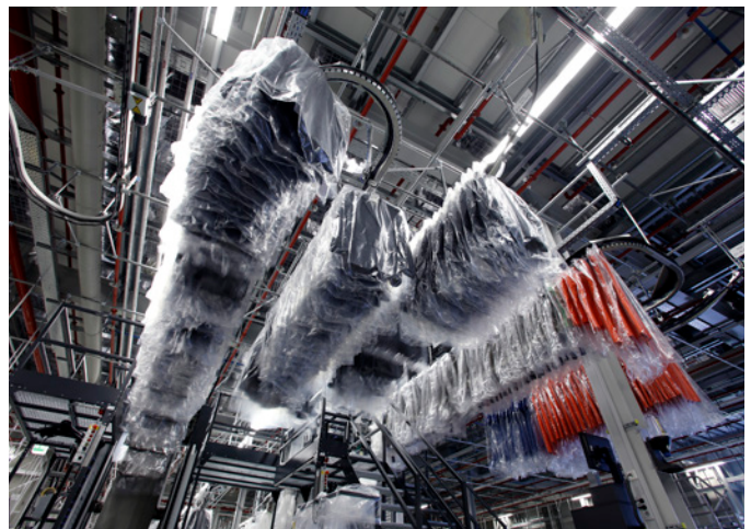
Use overhead space for storage and reserve floor space for actual work.
